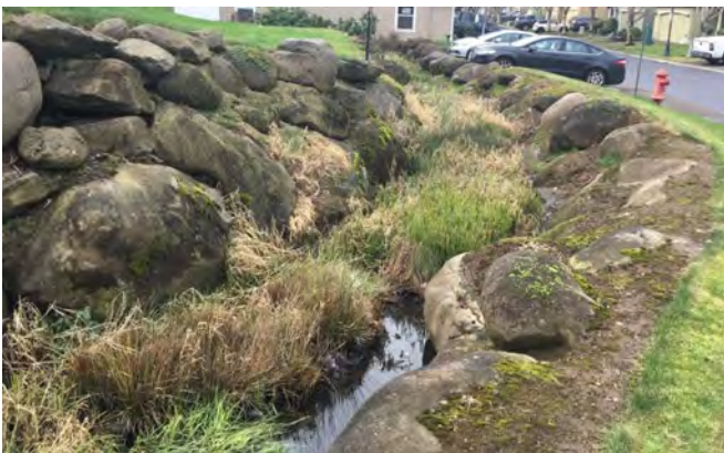
Below ~ Stormwater Planter
