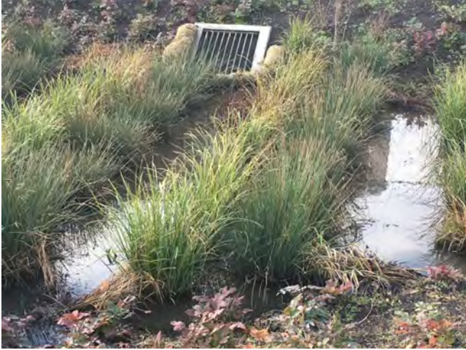
Above ~ Detention Pond
