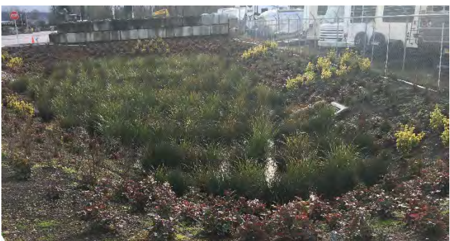
Below ~ Stormwater Planter
